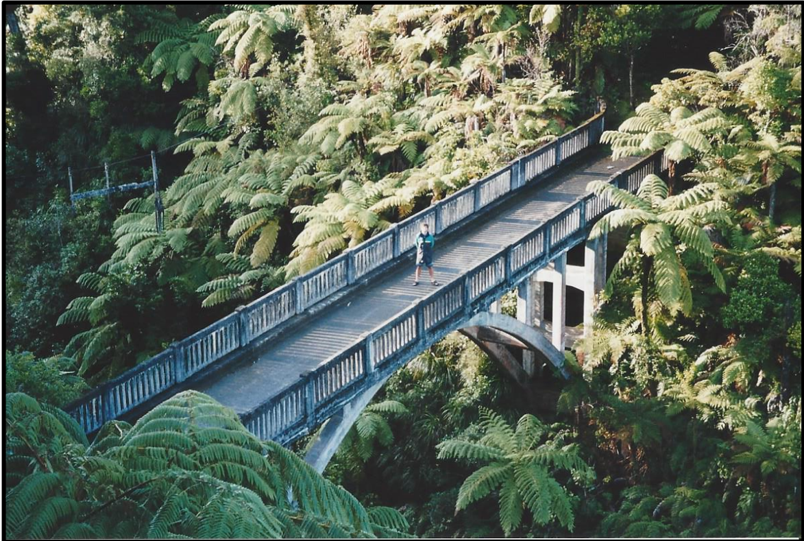
Bridge To Nowhere
